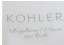
Gallons per flush are printed on toilet bowl or tank
