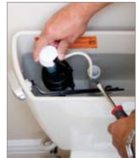
Fix toilet tank leaks
