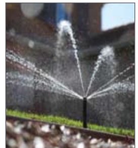
Replace sprinkler spray heads with MSMT nozzles.
