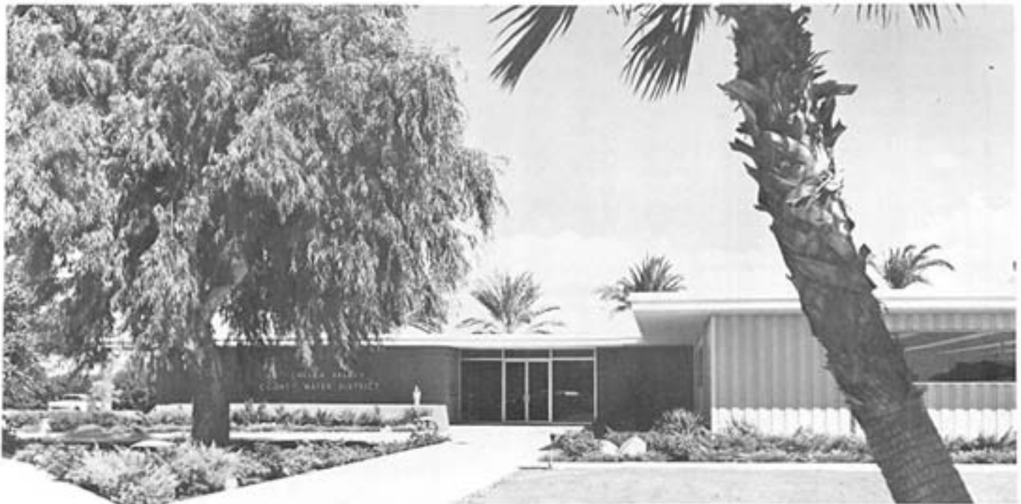
OUT OF ASHES ROSE THIS NEW DISTRICT HEADQUARTERS
