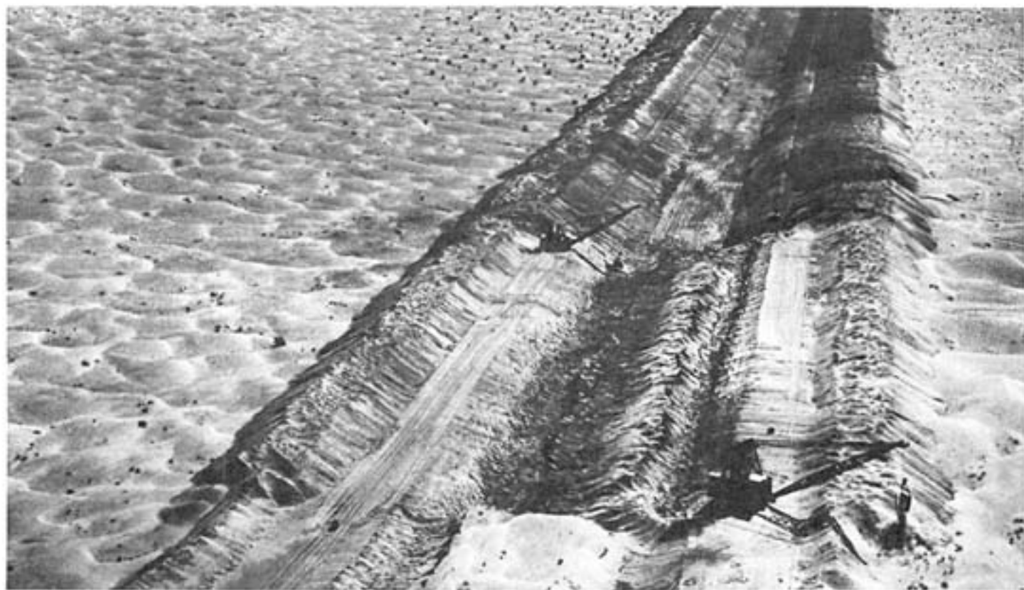
COACHELLA BRANCH ALL AMERICAN CANAL BUILDING BEGAN IN 1938
