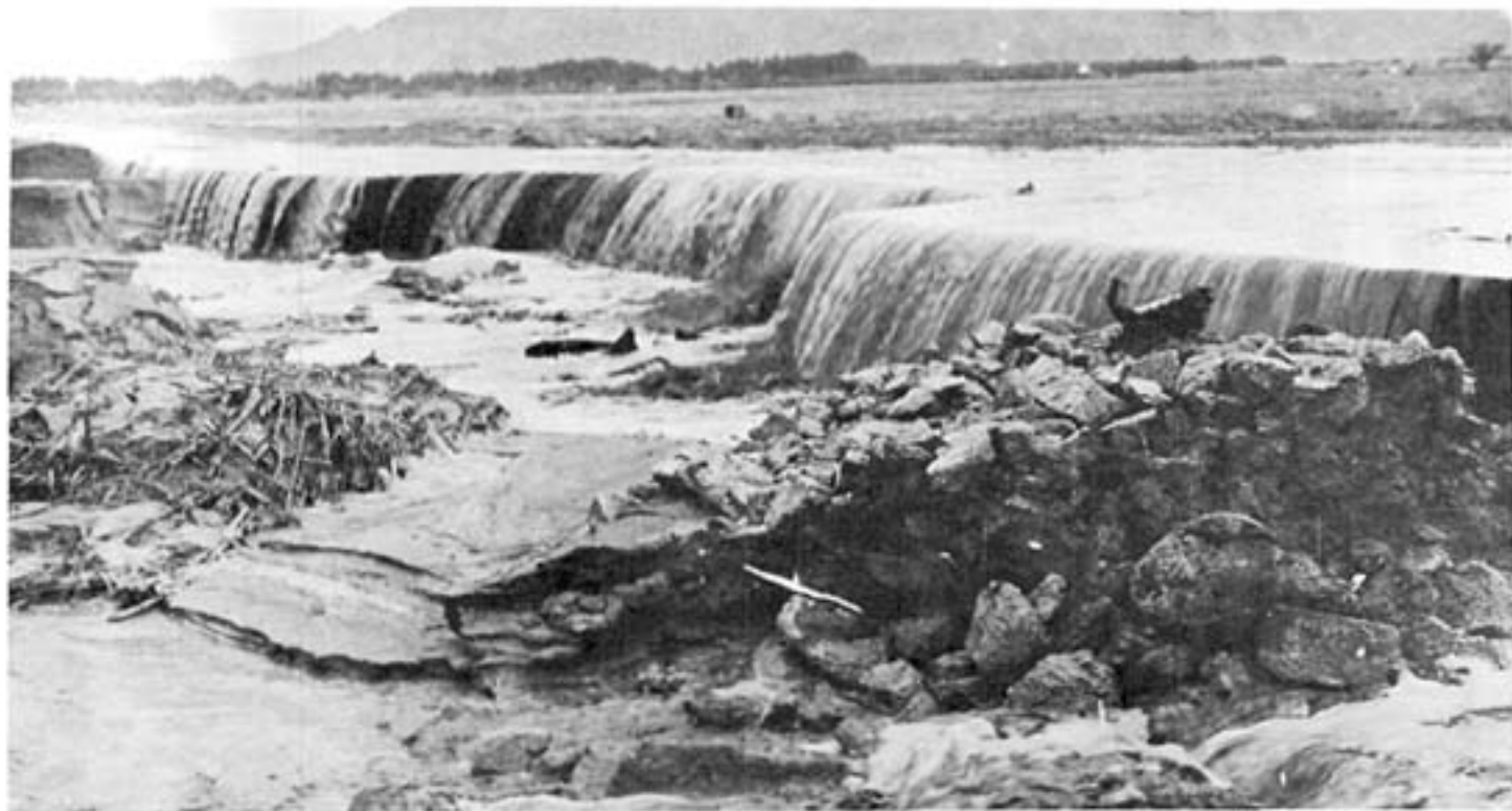
1927 DEEP CANYON FLOOD DAMAGED INDIAN WELLS AREA
