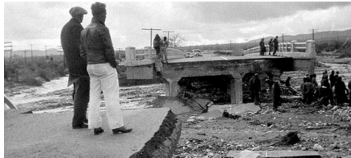
Men survey the washed out Palm Springs Bridge over Tahquitz Wash on Palm Canyon Drive after the 1938 flood. Courtesy of Coachella Valley Historical Society
