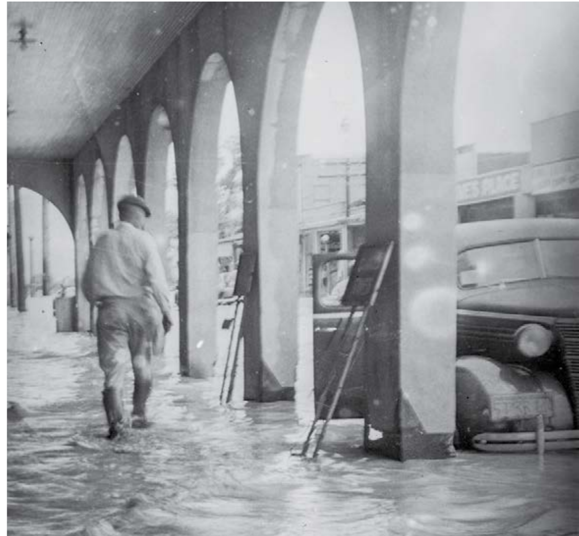
Flooding in downtown Coachella in 1939. Courtesy of the Coachella Valley History Museum
