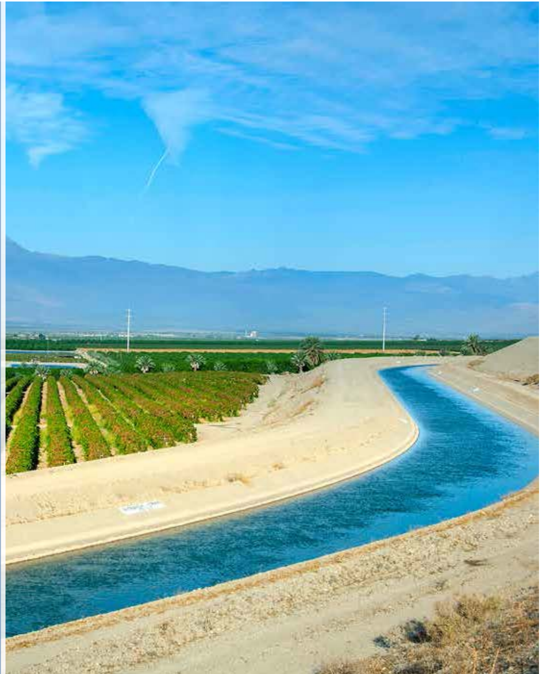
The Coachella Branch of the All-American Canal is one of two lifelines that bring Colorado River water into the valley. CVWD archive photo
