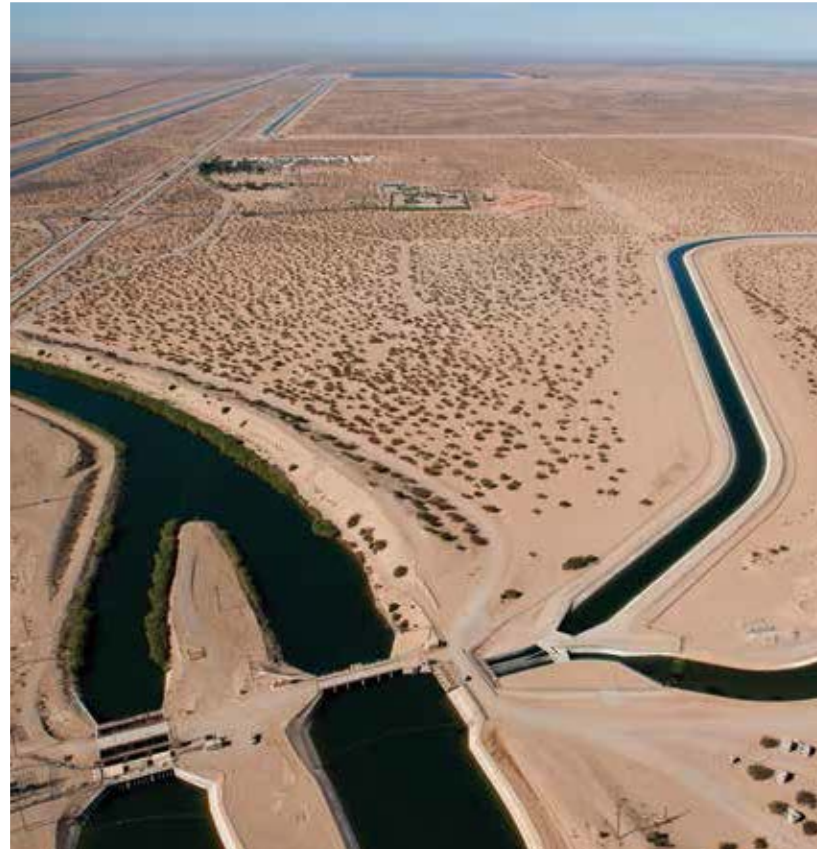
The drop turn-out of the All-American Canal leading to the Coachella Canal. The Coachella Canal is on the right. CVWD archive photo
