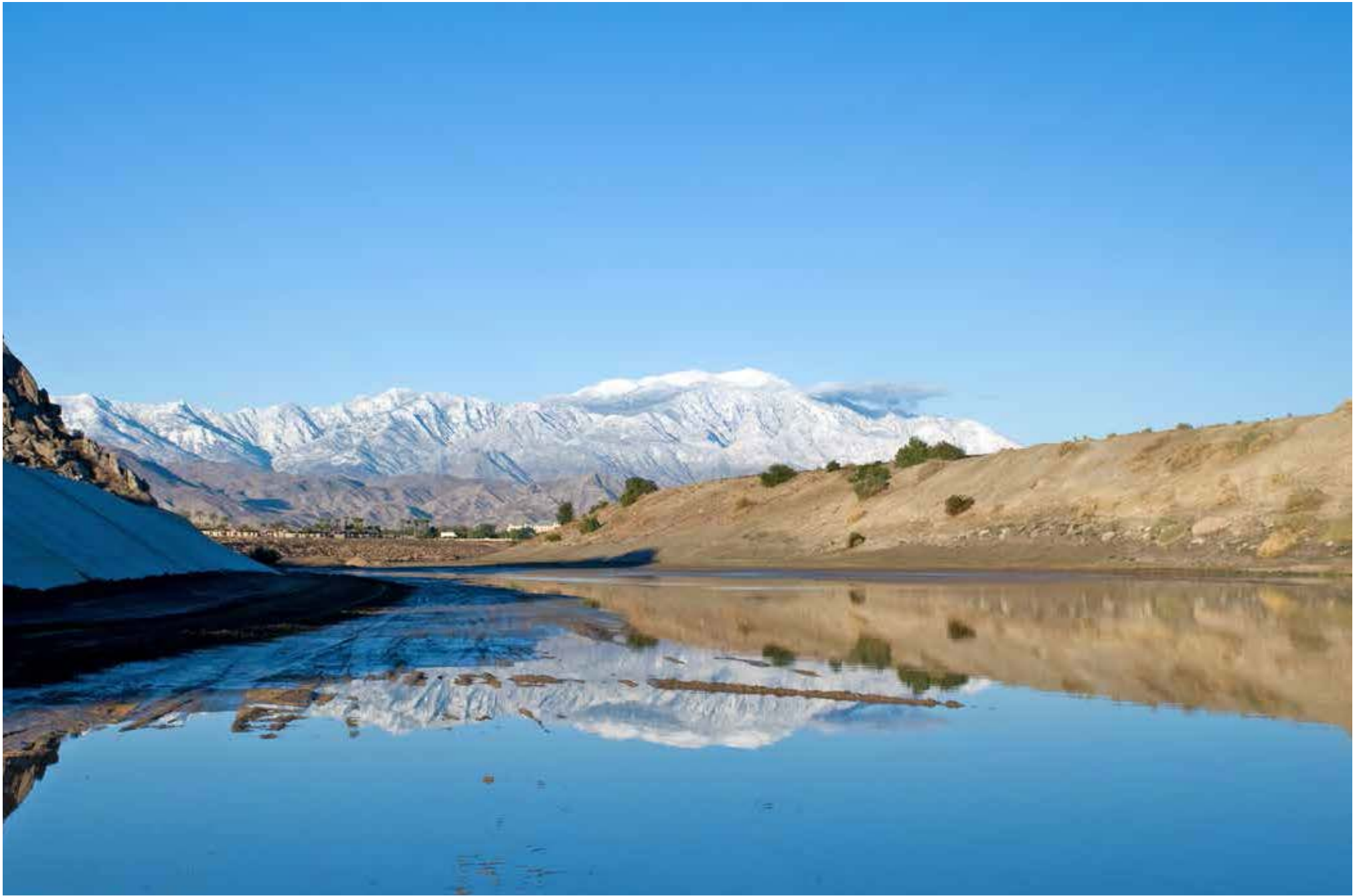
Whitewater Flood Control Channel at Point Happy in La Quinta. CVWD archive photo
