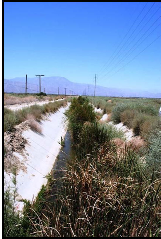
Figure 2 Concrete Lined Agricultural Drain at Southern End of Parcel
