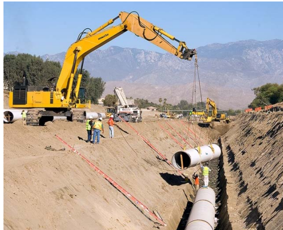
Construction of the Mid-Valley Pipeline
