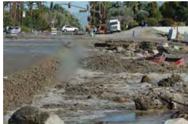
CVWD's Stormwater Facilities Provide Flood Protection
