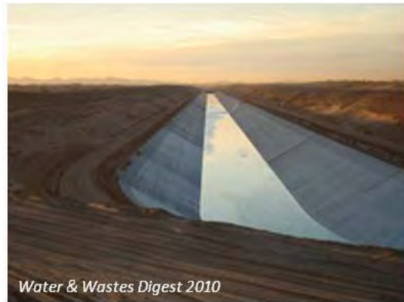
Coachella Canal Lining Project
