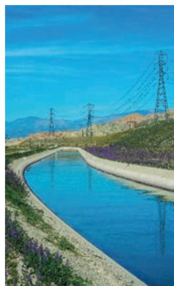
The Coachella Canal was completed in 1948, with CVWD taking water delivery in 1949. Water that flows through the Canal travels several hundred miles, via gravity flow. It starts at the Colorado River and diverts into the All American Canal at the Imperial Dam, located 18 miles north of Yuma, Arizona. The water is diverted again, 38 miles downstream, into the Coachella Canal.
