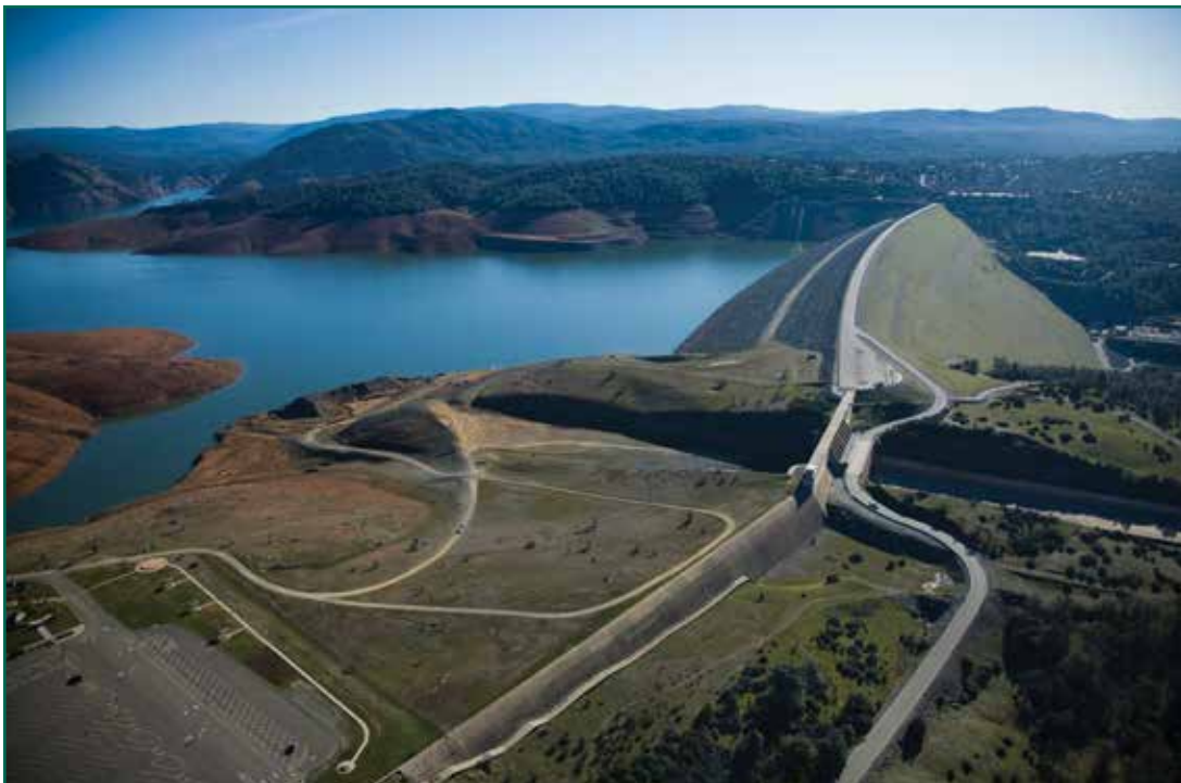
Oroville Dam Spillway
