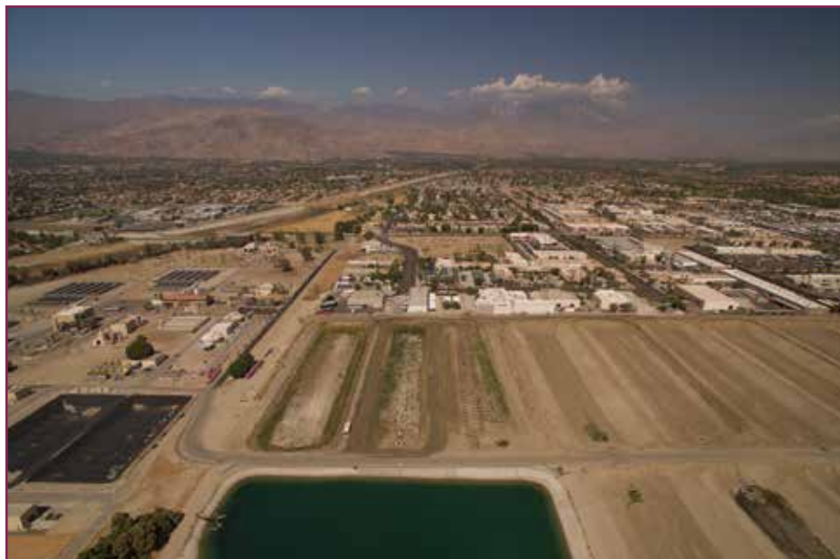
Aerial view of Wastewater Reclamation Plant No. 10 with location of upcoming replenishment facility
