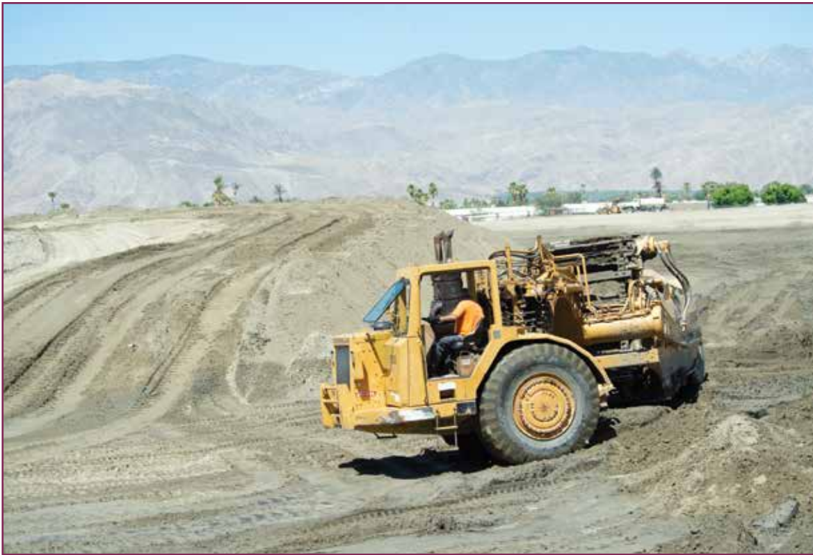
Grading for the new Groundwater Replenishment Facility in Palm Desert
