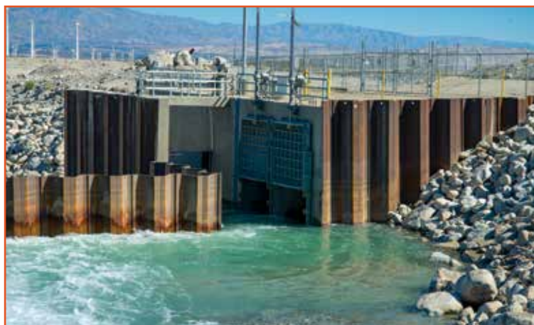
Diversion intake structure at the Whitewater Replenishment Facility
