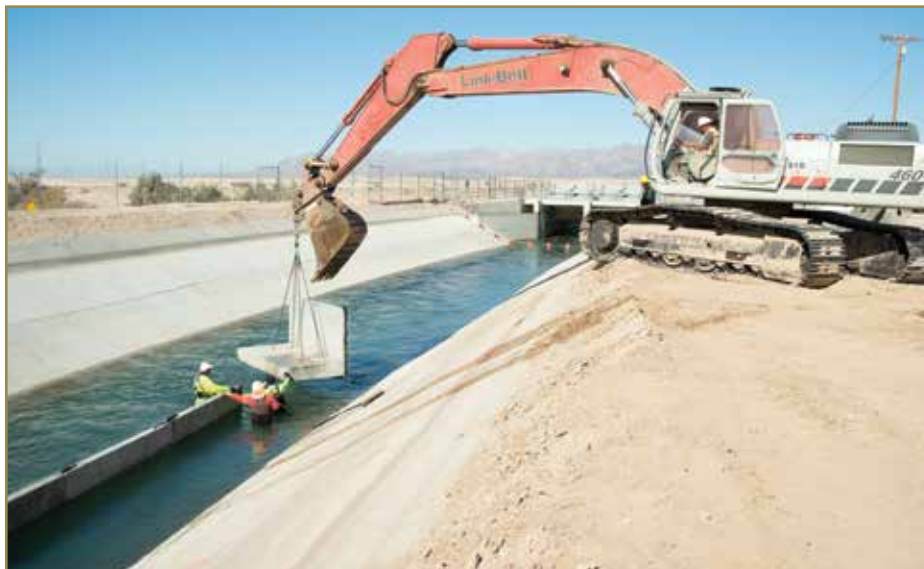
Repairs on the Coachella Canal
