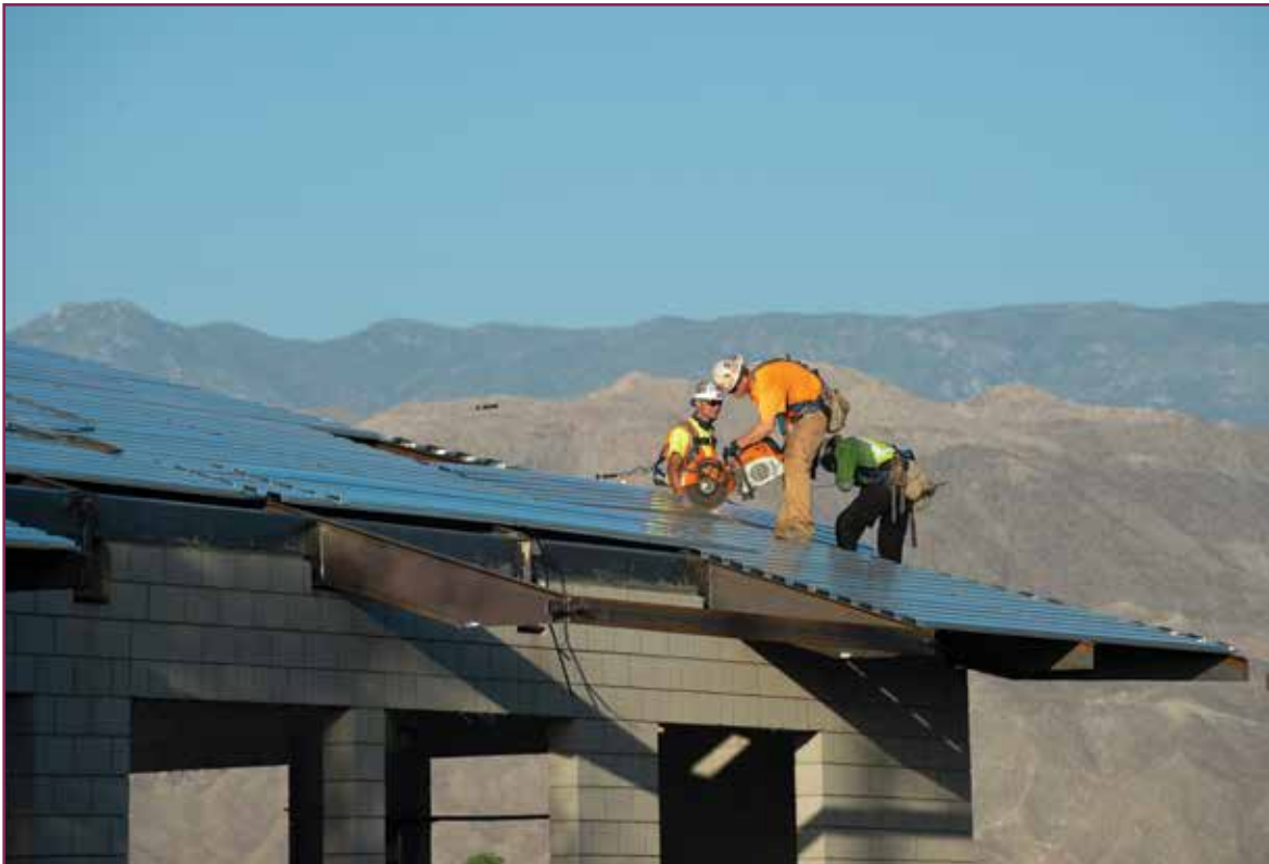
Construction of the new Critical Support Services Building in Palm Desert
