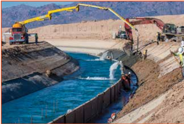
Lining repair on the Coachella Canal
