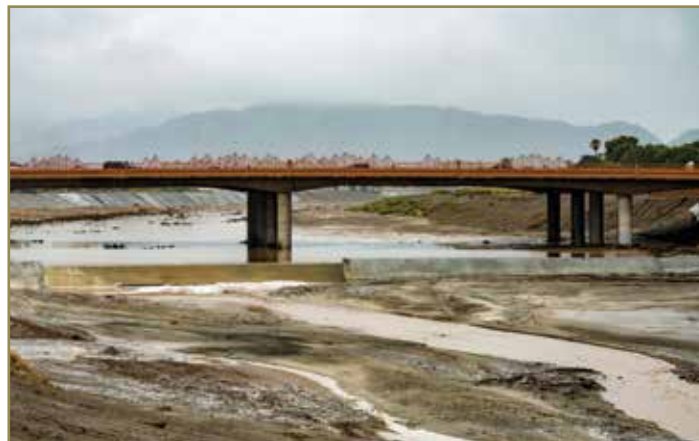
Whitewater Stormwater Channel
