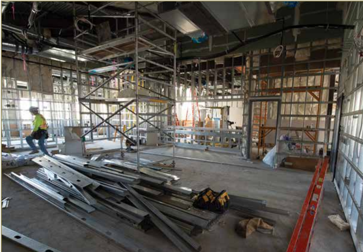
Critical Support Services Building under construction
