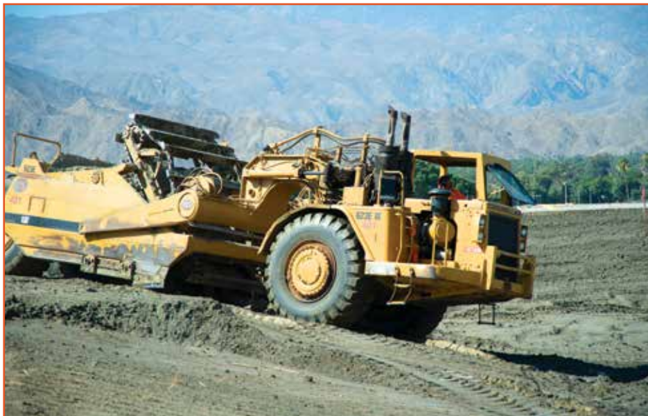
Grading for the new replenishment facility in Palm Desert
