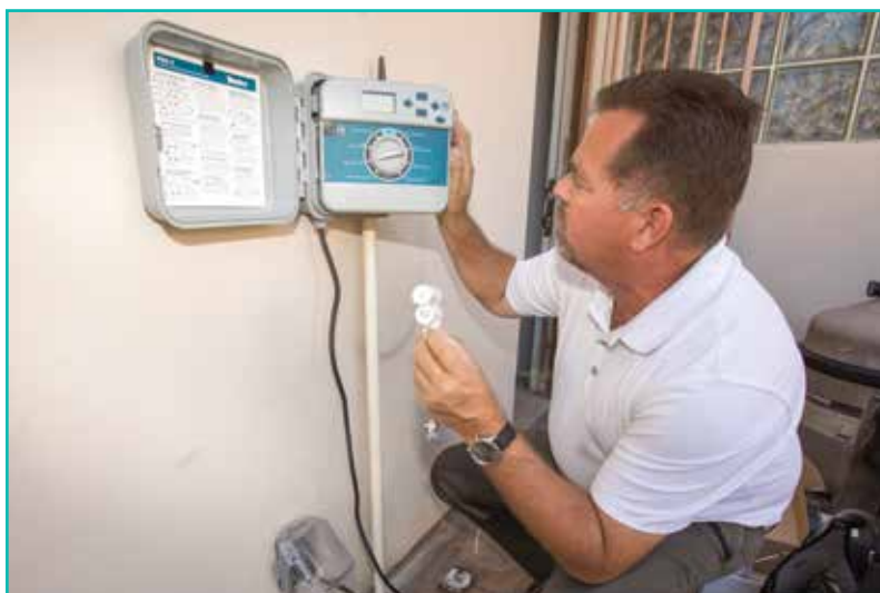
Installing a Smart Controller
