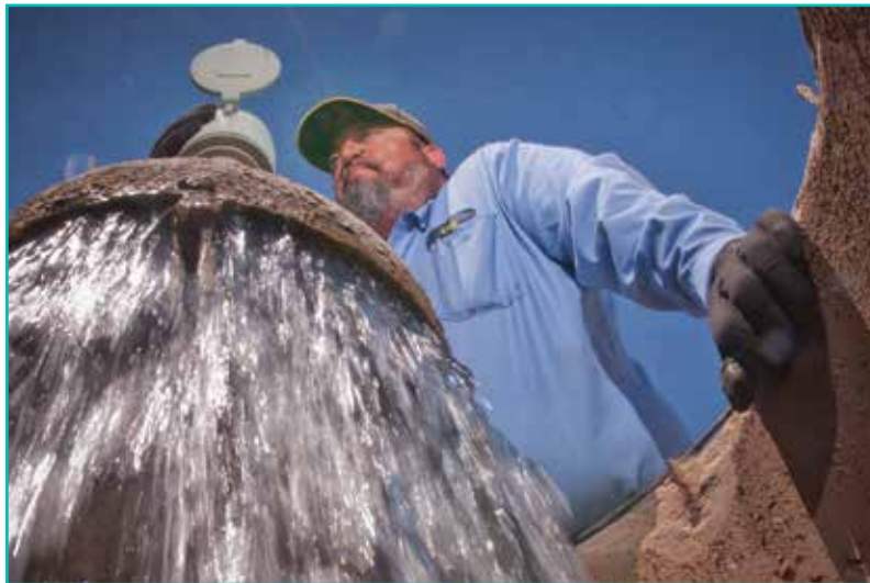
Zanjero checking the reading on a flow meter at a CVWD delivery point
