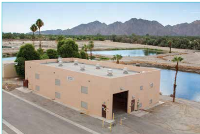
Chlorine Building at WRP 10
