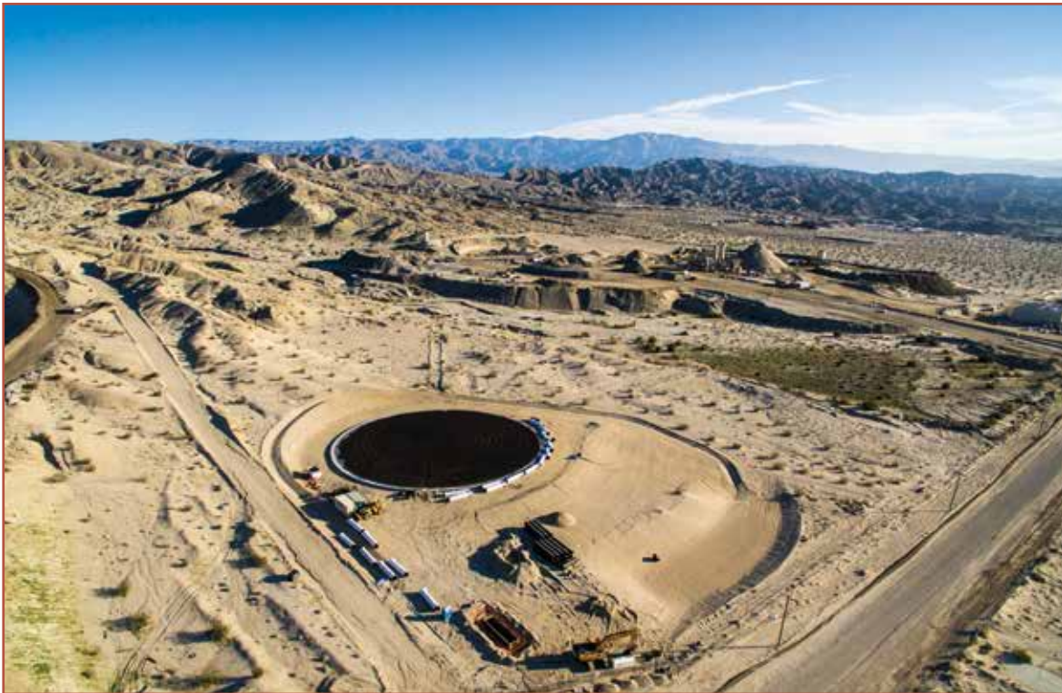
Reservoir under construction in Thousand Palms, CA
