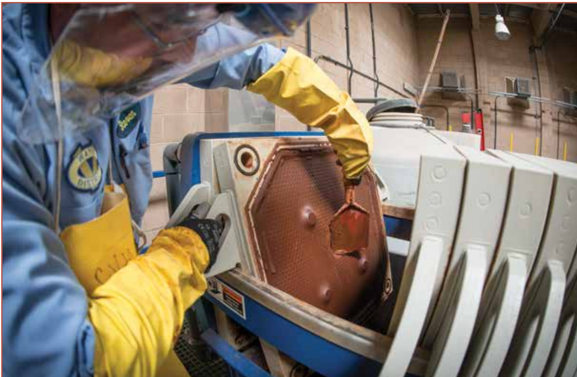
At the Ion Exchange Plant in Thermal, CA, crews clean pressure plate filters of red waste material.
