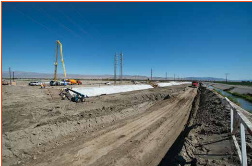
Fillmore Street Irrigation Ditch Project
