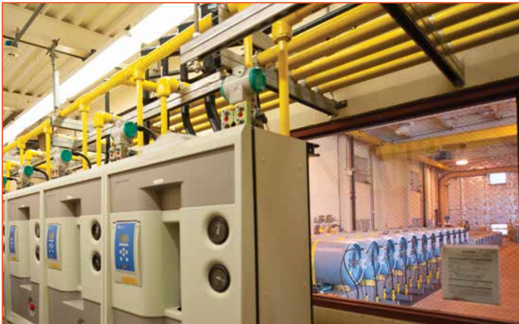
Chlorine room upgrade at WRP 10
