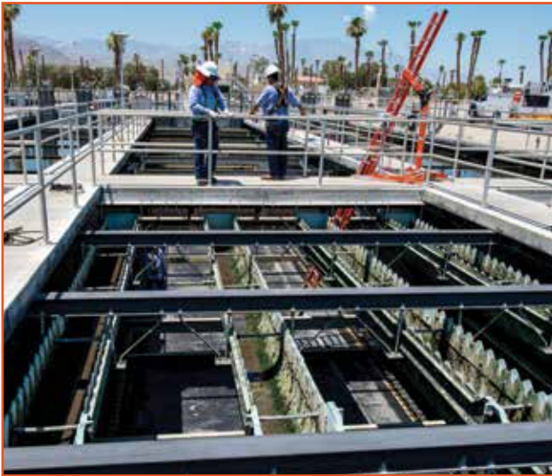
Clarifier repairs at WRP 10
