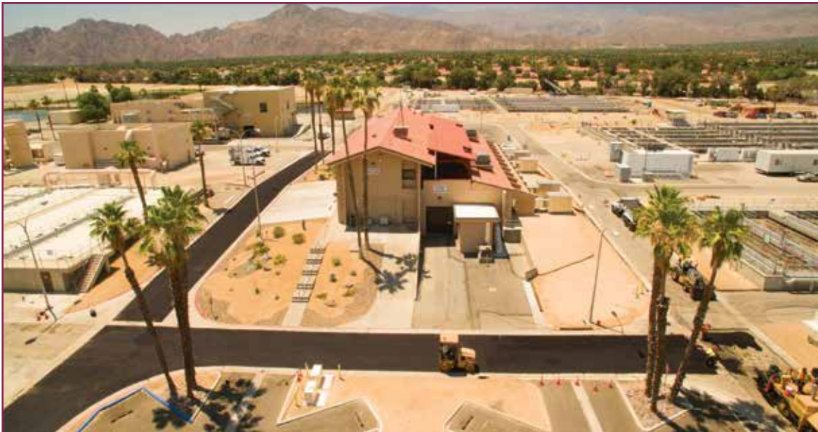
Paving project at WRP 10
